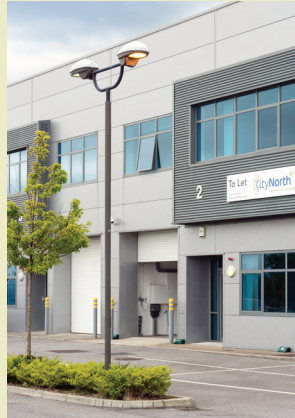
Unit 2 - external view
