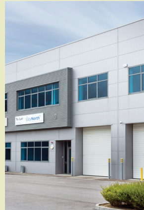
Unit 3 - external view
